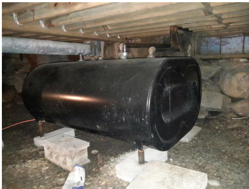
Figure 1 – Existing Oil Tank
