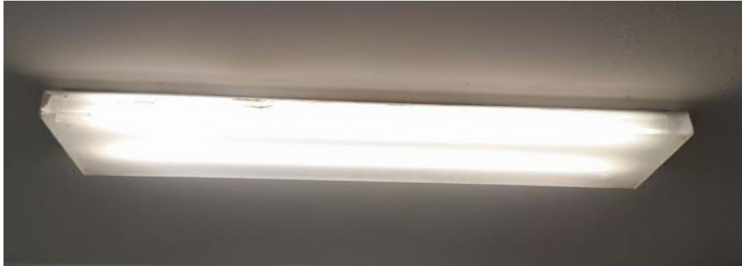
Figure 22 – Existing Ceiling Mounted Wrap
