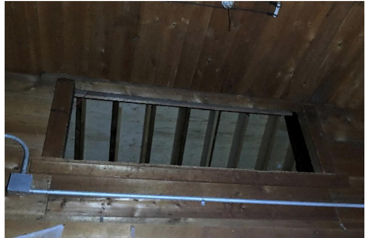
Figure 8 – One of the many hatches open to the attic
