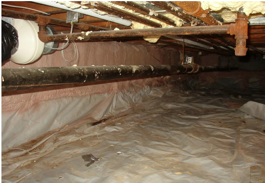
Figure 6 – Fully installed Tu-Tuff and spray foam.
