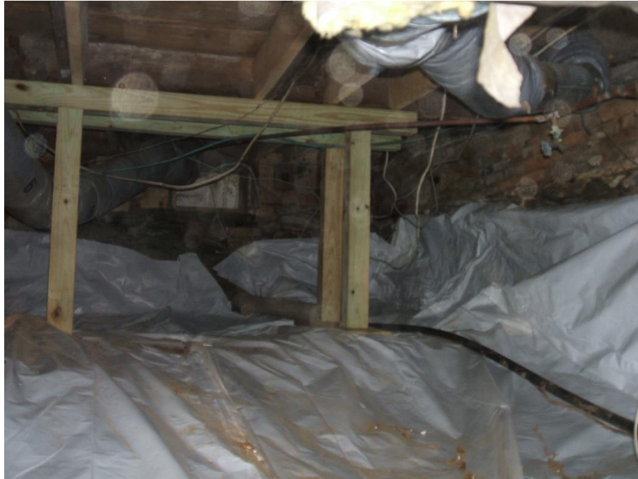
Tu-tuff lapped up onto walls prior to spray foam install.
