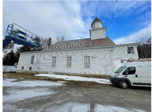
Figure 10 – The walls as viewed from outside.
