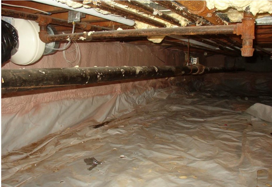
Fully installed Tu-Tuff and spray foam.
