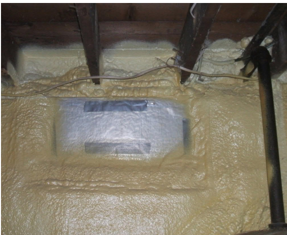
Figure 4 – Spray foam and window infill
