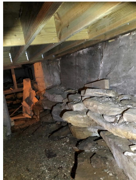
Figure 3 – The stone foundation is visible from within the crawlspace.
