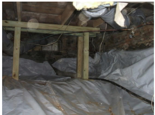
Figure 5 - Tu-tuff lapped up onto walls prior to spray foam install.
